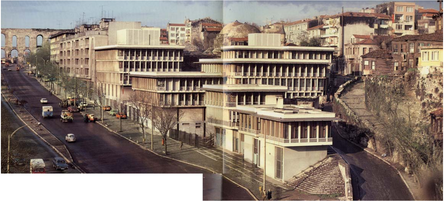
FIG.1. The resulting structure is tied to the context in a manner that conceals the actual limitation of the lot.
